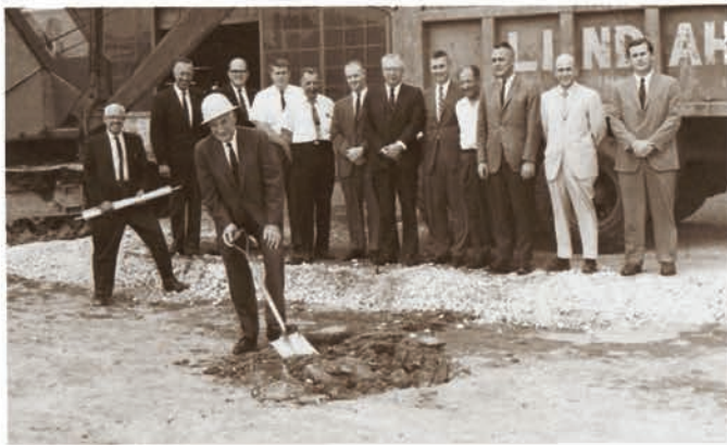
Breaking Ground For Addition At Armstrong Avenue Plant, 1967
