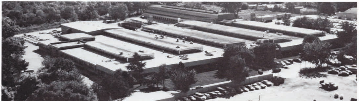
Plant at Armstrong Avenue
