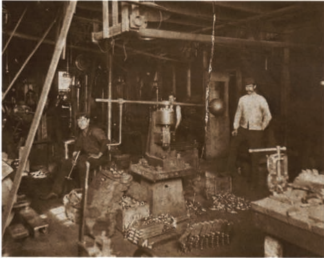
Early Plant Photo
